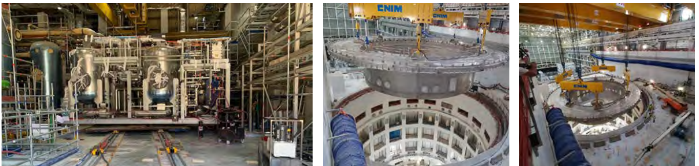
Numerous special EUROPRESS cylinders and power packs have been vital for the operations of shifting and correct positioning of the structural parts of the Tokamak, the beating heart of the ITER reactor. San Paul Les Durance, France.
