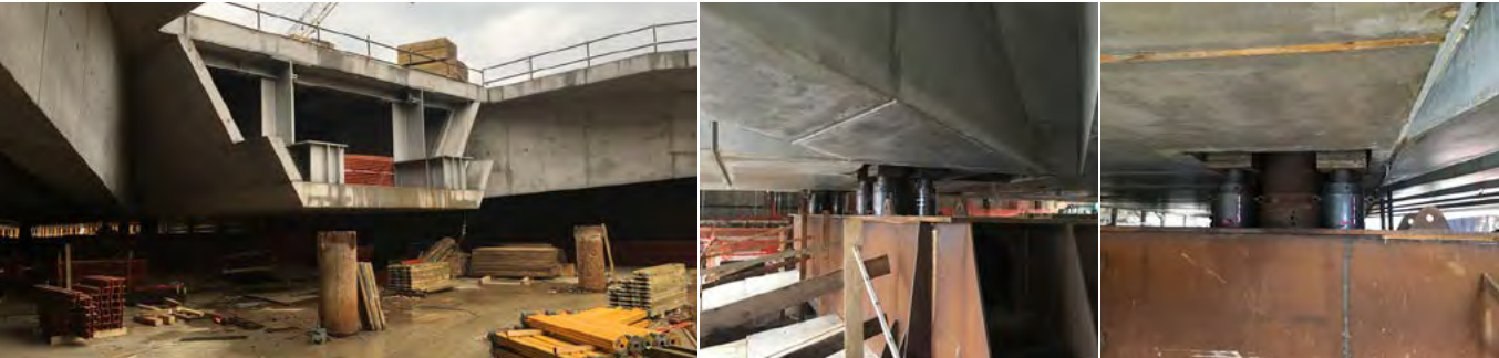
Positioning of the roof insole in the new high speed Belfiore station with the help of ME power packs and CGG cylinders. Florence, Italy.
