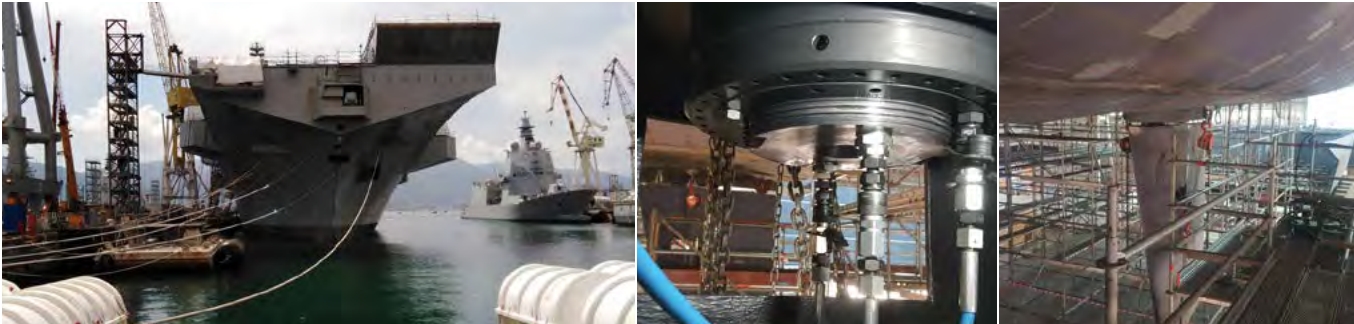
Fastening of the rudder blades on the respective rods with hydraulics nuts and 1500 hydraulics power packs. Doha, Qatar.
