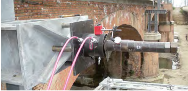
COF Hollow ram cylinders for anchor bars stringing on a railway bridge.
