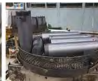
Phase 8 Washing and cleaning of the components which will be ready to be assembled.
