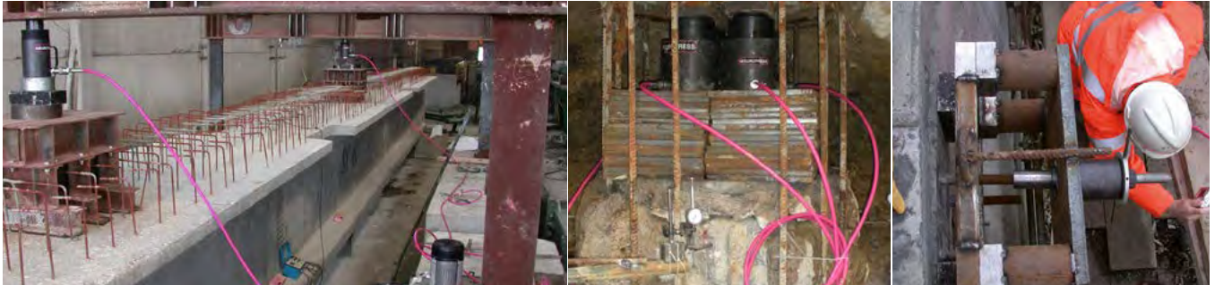
Deflection test on prestressed beams with Europress big tonnage cylinders and power packs.
